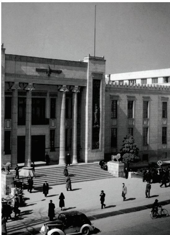
Figure 4. The central building of Melli Bank in old Tehran.
